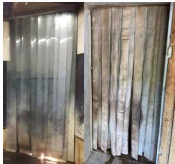
Figure 27: Lamella for minimising temperature loss, made out of plastic or fire hose. © Paris Zoo, D. Koch
